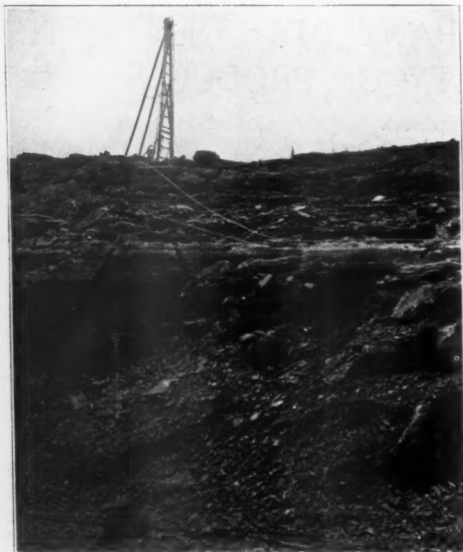
Drill at Top of Quarry
